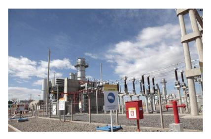
Loma Campana Este is located 16 km from the Loma Campana Complex. It is made up of 12 natural gas engines with a total capacity of 17 MW. This plant supplies energy to the 13.2 kV Unconventional Field called Loma Campana.
